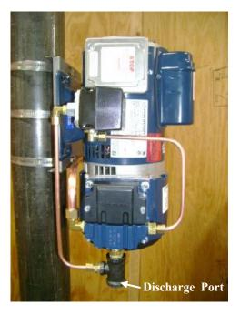
After the mounting plate is properly mounted on the riser, secure the compressor to the plate using the compressor hooks to temporarily hold the compressor in place. Then use all four (4)nuts, washers and bolts to permanently mount the compressor to the plate. **Straps must be 90° angle to riser for proper installation.**
