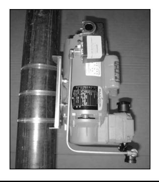
Once the straps are threaded in the holes and the compressor is bolted to the plate, secure the compressor and plate to the riser using the straps as shown here. **Straps must be 90° to riser for proper installation.**
