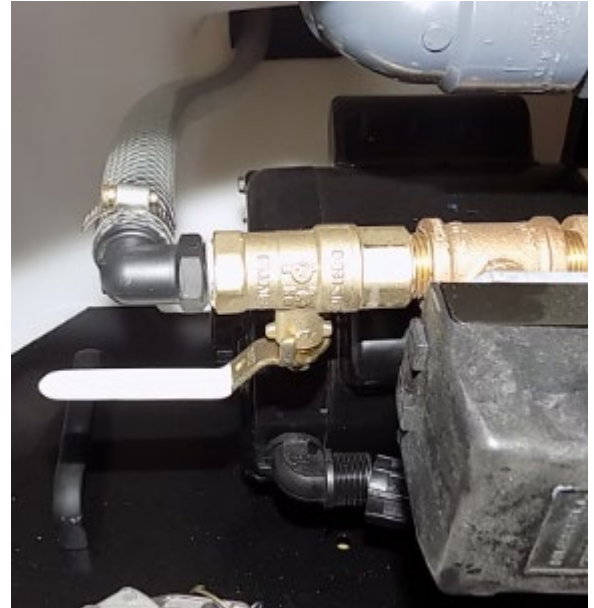
Open position: ball valve and handle form an "I" shape
