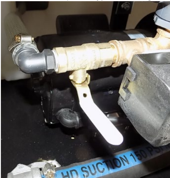
Closed position: ball valve and handle form a "T" shape
